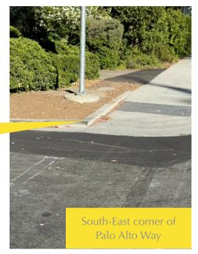
This sharp 90° curb corner has a high likelihood of causing tire and wheel damage, leading to tire failure. It seems that a rounded or ramped corner would be safer and less damaging.
