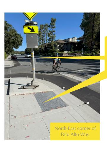
The crosswalk ramp fails to accommodate disabled persons by placing the crosswalk button out of reach and on the opposite side of the pole
